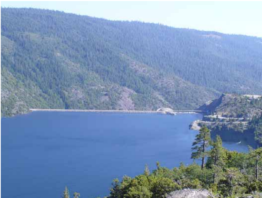
Sim 2 - Existing structures with 6-foot raise in current maximum normal operating WSE, Plus new spill way gates. (Note that neither the new or existing power lines are discernable from this KOP.)
