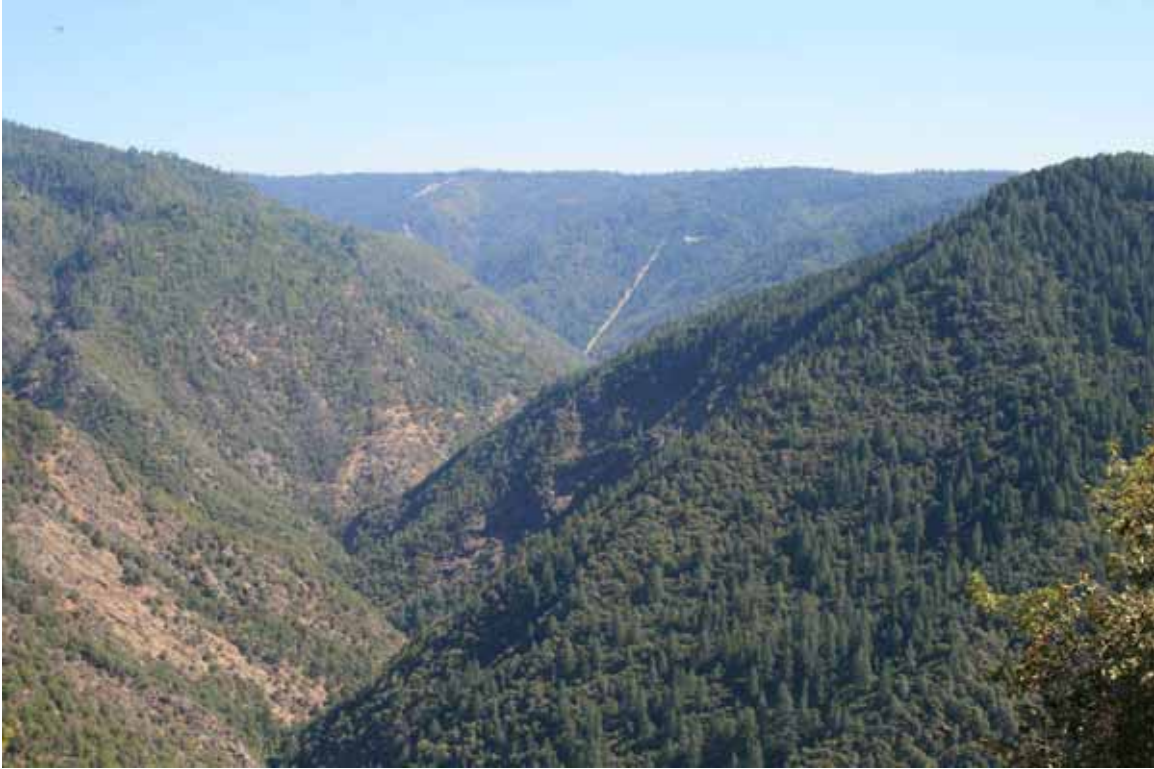
Photo 3. View of Middle Fork Powerhouse Penstock from Mosquito Ridge Road near Dutch Flat.
