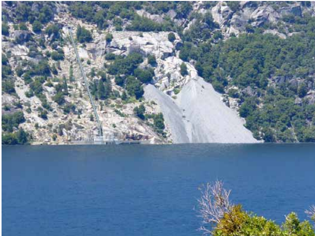
Sim 4 - Existing structures with 6-foot raise in current maximum normal operating WSE.
