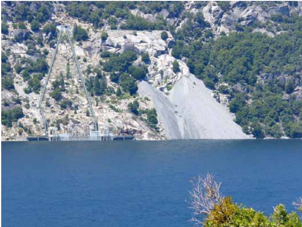
Sim 8 - Existing structures plus new structures with current maximum normal operating WSE.
