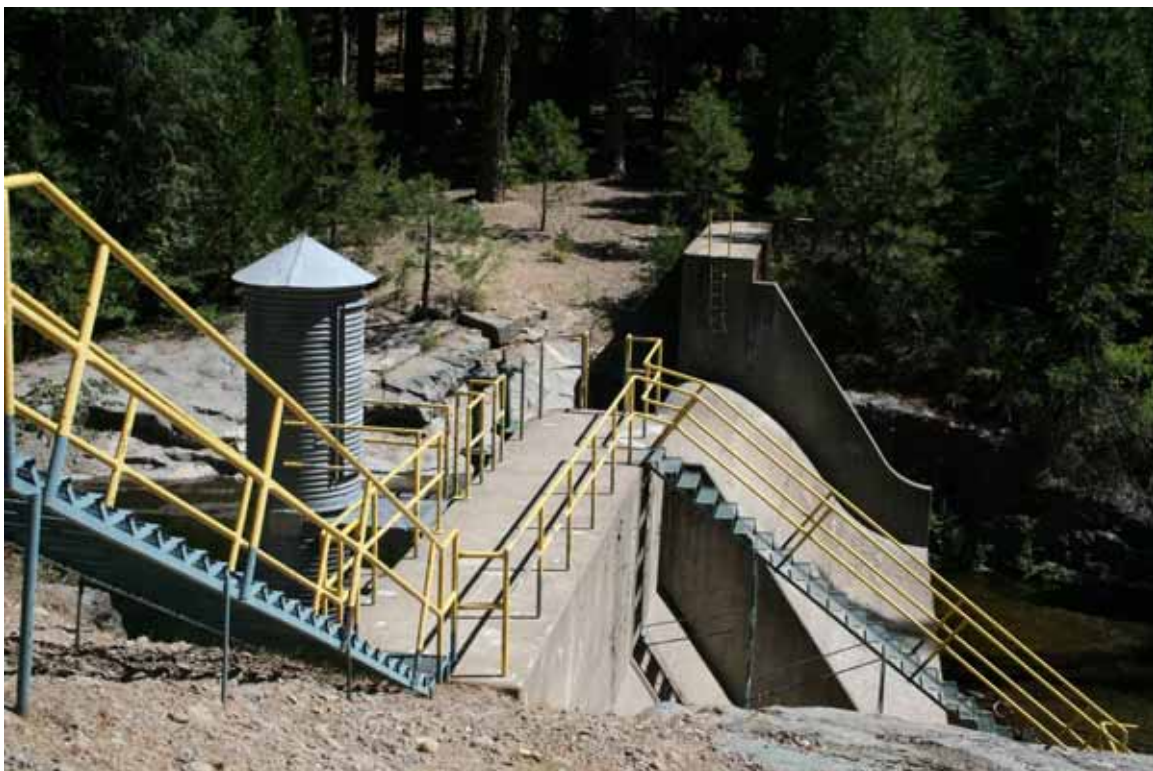
Photo 19. View of South Fork Long Canyon Creek Diversion from above the creek.
