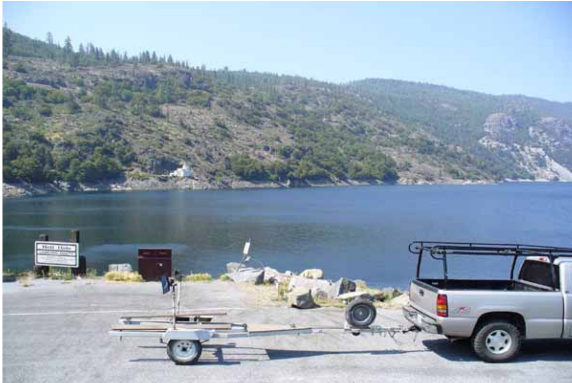
Photo 20. View of Hell Hole Gatehouse (in foreground) and French Meadows Powerhouse (in background) taken from Hell Hole Boat Ramp Parking Area.
