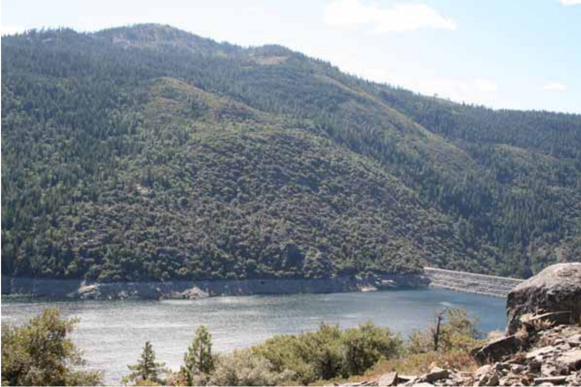
Photo 22. View of Hell Hole Dam from edge of Hell Hole Campground looking south.
