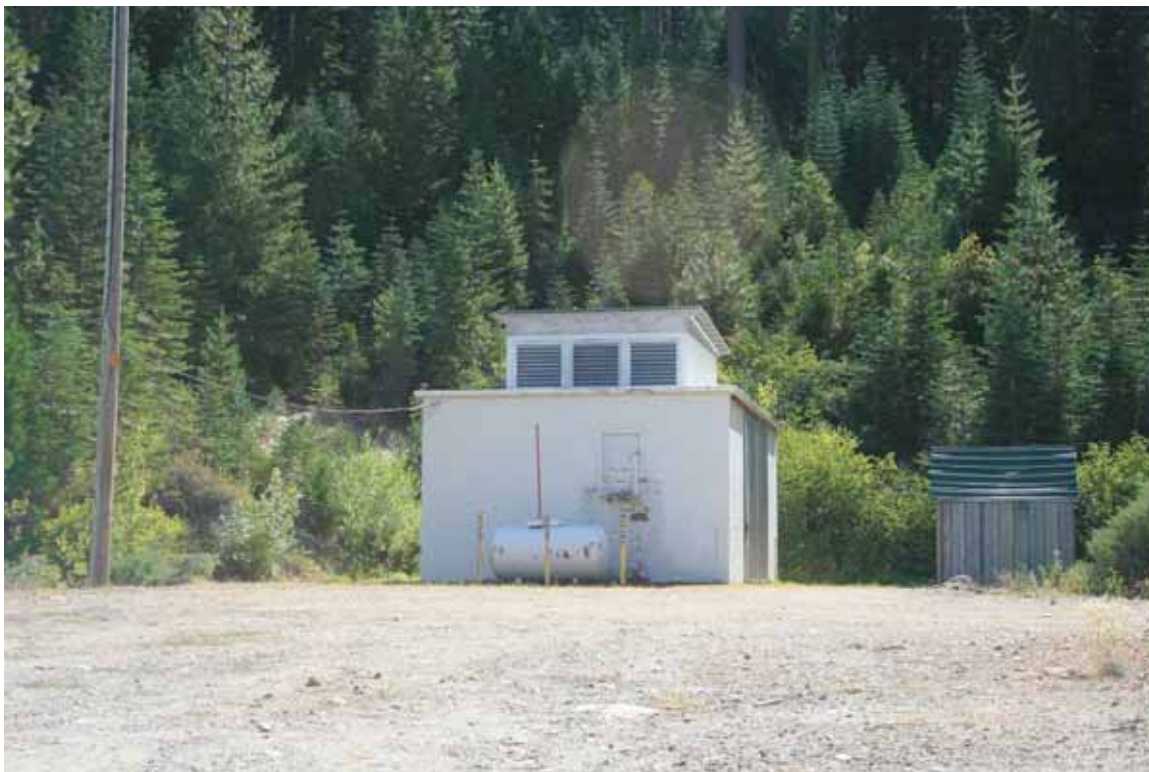
Photo 7. View of French Meadows-Hell Hole Tunnel Gatehouse from French Meadows Reservoir viewshed.
