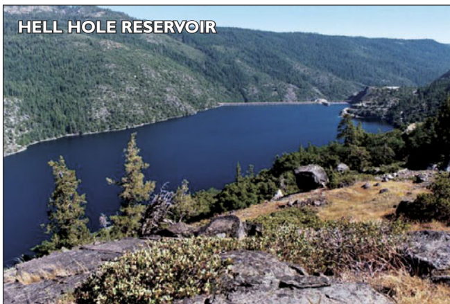
Installation of spillway gates on Hell Hole Reservoir will increase seasonal storage and power generation.
