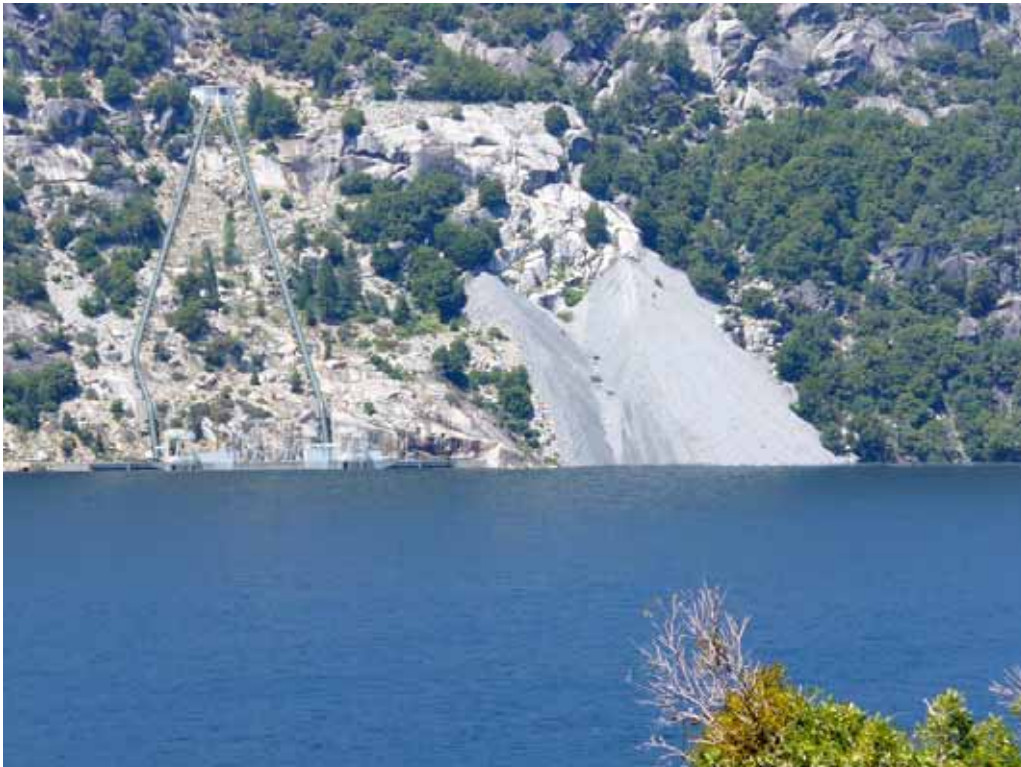
Sim 12 - Existing structures plus new structures with 6-foot raise in current maximum normal operating WSE.
