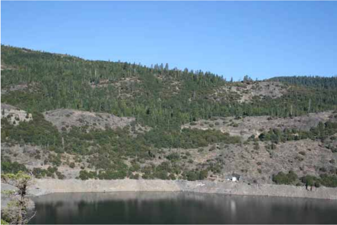
Photo 16. View of Hell-Hole - Middle Fork Tunnel Gatehouse from Upper Hell Hole Trail (Hell Hole Reservoir viewshed).
