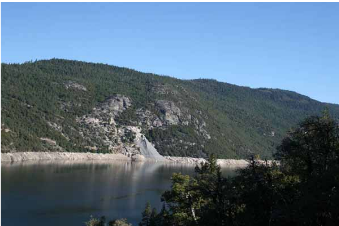
Photo 15. View of French Meadows Powerhouse and Switchyard area from Upper Hell Hole Trail (Hell Hole Reservoir viewshed).
