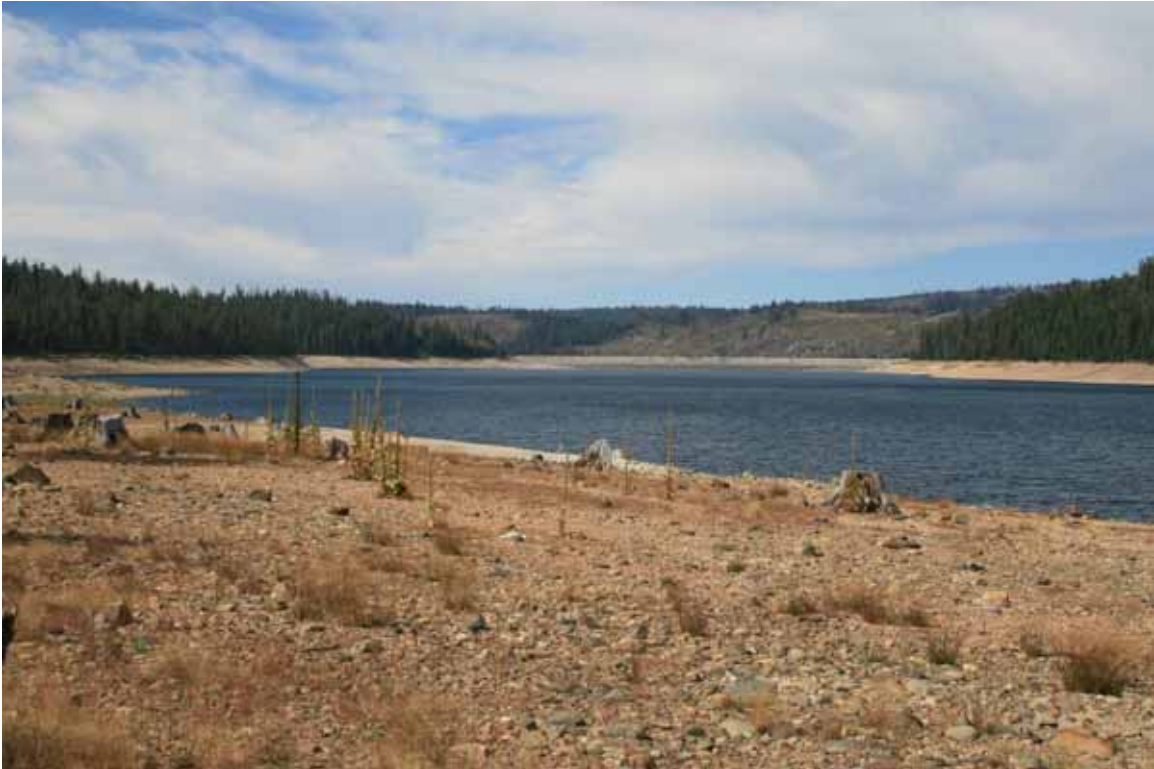
Photo 11. View of French Meadows Dam looking west from French Meadows Boat Ramp.
