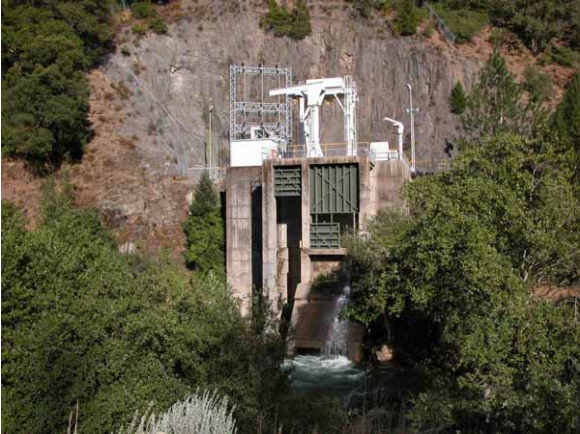
Photo 13. View of Oxbow Powerhouse and Switchyard from near the Indian Bar Rafter Put-in.
