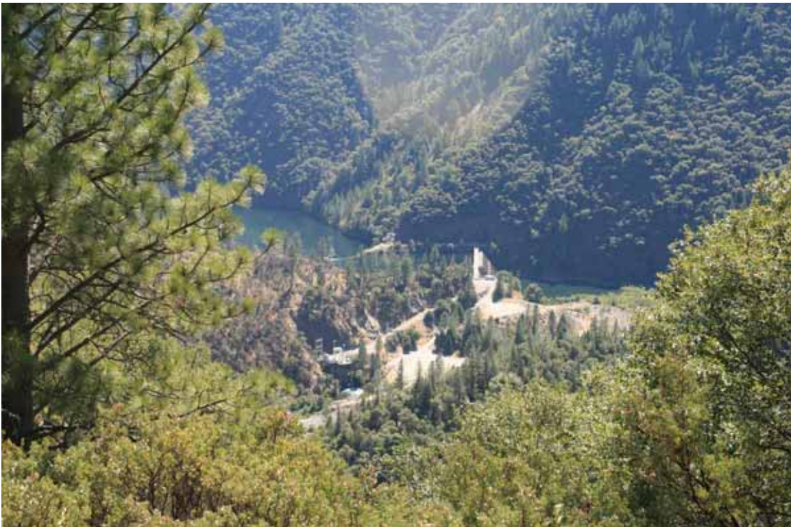
Photo 2. View of Ralston Afterbay Dam and associated features from Mosquito Ridge Road.
